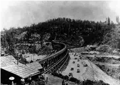
Figure 4.6 Chinese laborers working on construction of railway bridge, circa 1880
