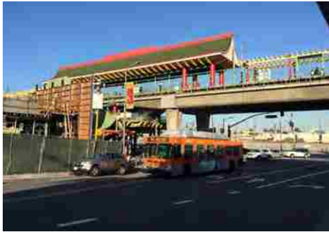
Figure 5.1.22 Metro station in Chinatown
